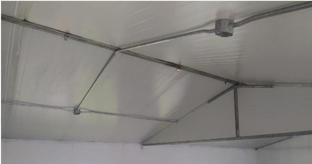
**FIGURE 4. TUBERÍA EMT DE 1/2 "INSTALADA CON CAJETINES OCTOGONALES**
