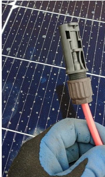
Figura 60: Conector MC4 anclado al conductor
