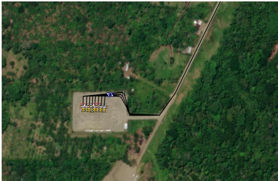
Figura 9: Well Pad SHSO
